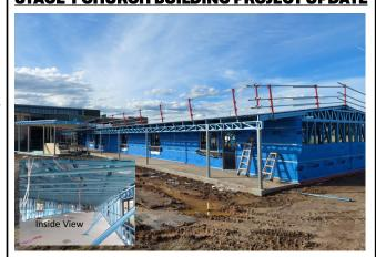
Installation of the roof and placing of frame sheeting in preparation for cladding.
